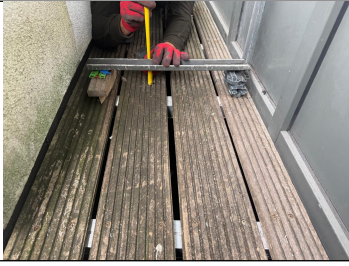
E3 - Weathering and decking joist replacement complete
